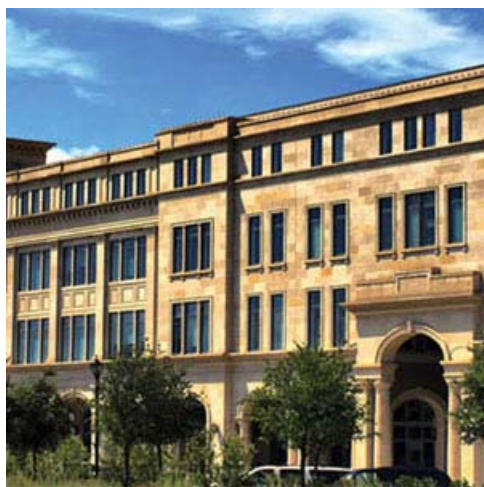
Five Star Development is using Condor SS to treat Frisco Square, a master-planned, multi-generational development near Dallas.
